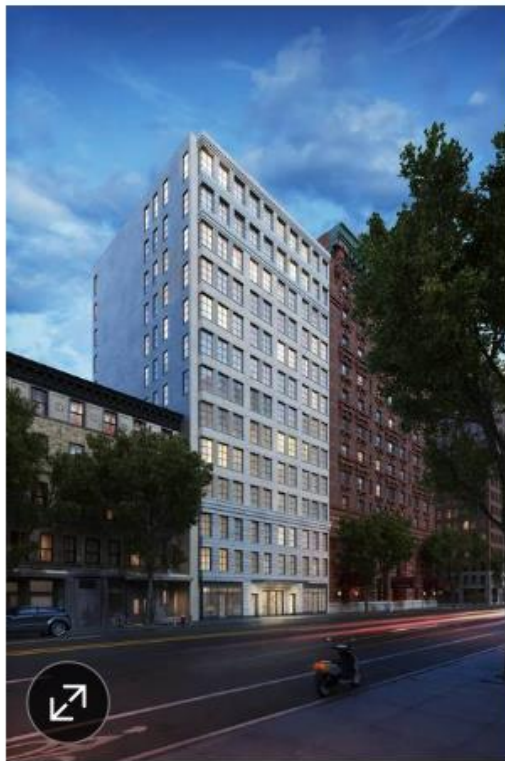
207W79, also under construction on the Upper West Side PHOTO: MOSO STUDIO
